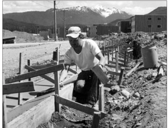
▲ Construction worker pours concrete for sidewalks in 1956 Kitimat.
