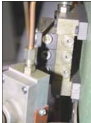
▲ The divider valve installed on air compressor 2 in building 140.
