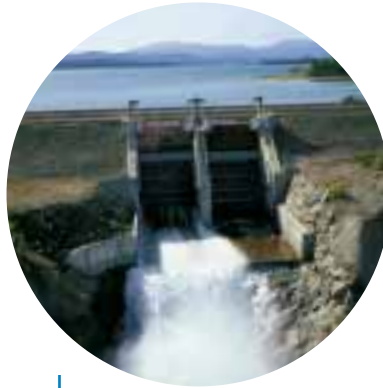
The Skins Lake Spillway is situated 80 km west of Kenney Dam and releases water from the Nechako Reservoir into the Nechako River by way of the Murray/Cheslatta system.
