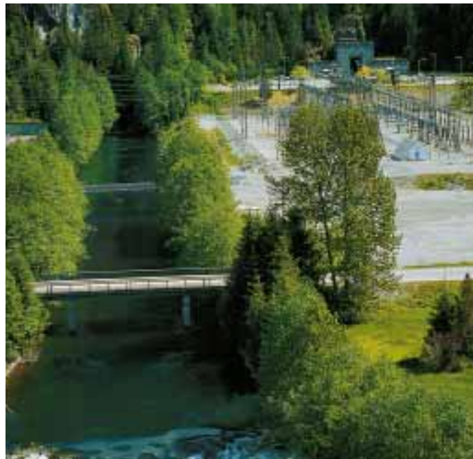
Water exits the Kemano powerhouse through a "tailrace" into the Kemano River.
