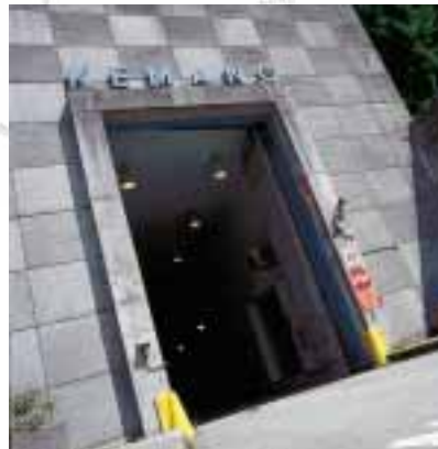
The Kemano powerhouse is a 1,000 megawatt hydroelectric generating station built inside the base of Mount Dubose.
