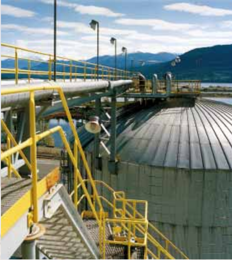
Kitimat Works' liquid pitch storage facility was built in 1997-98, at a cost of $14 million, to enclose pitch handling and eliminate pitch losses.
