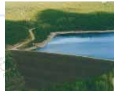
The Kenney Dam impounds the waters of the Eutsuk/Tahtsa drainage basin.
