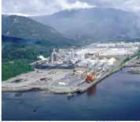
Kitimat Works is a 272,000-tonnes-per-year aluminum smelter located on the north coast of British Columbia, at the head of Douglas Channel. Kitimat's deep sea port enables the import of raw materials and export of value-added aluminum ingot.
